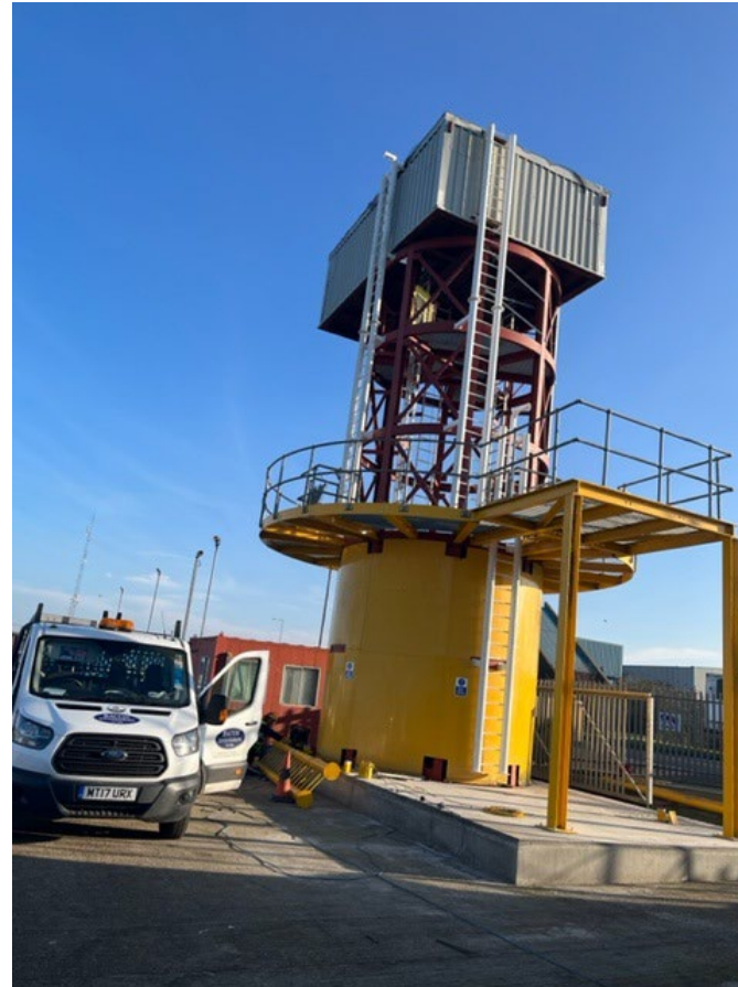
Offshore Training Centre (OTC) Turbine Training Tower in Grimsby
