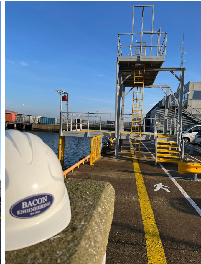
Offshore Training Centre (OTC) Training Platform in Grimsby
